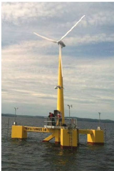
Figure B-2. Semi-submersible FOWT (VoltturnUS 1:8-scale) (left panel) and its structural components (right panel) (figure from Viselli, 2015).
