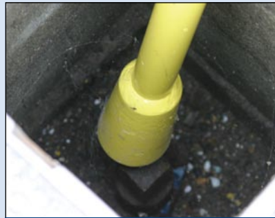
Fits over sluce valve spindle
